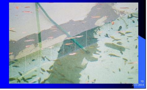
. A hose left in a pool is considered a cross connection because of the potential for the pool water to travel back up the hose, especially if there is no vacuum breaker on the hose bib. Vacuum breakers are easy to install, cheap, and are another very effective way to prevent backflow. Don't leave hoses in the pool!
