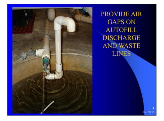
An air gap is the one of the most effective way to prevent cross connection and backflow. Provide air gaps on autofill discharge and waste lines to keep any potentially contaminated water from going back up into the system.
